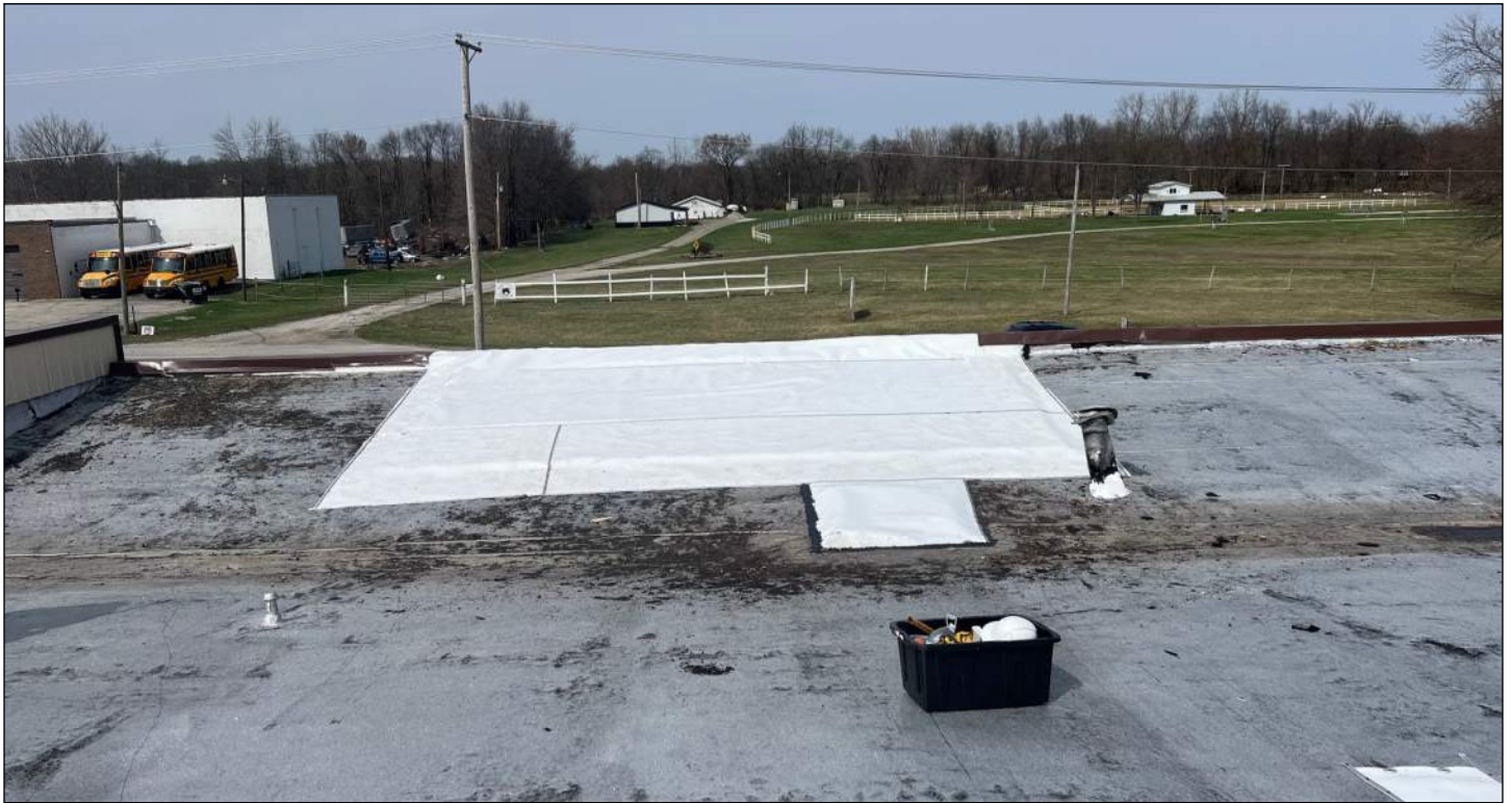
Image 7: Overview of roof after installation of temporary covering.
