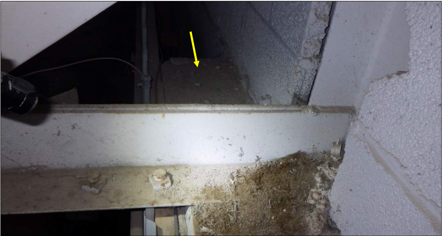
Photo 55: CMU pilaster (arrow) at truss bearing location.
