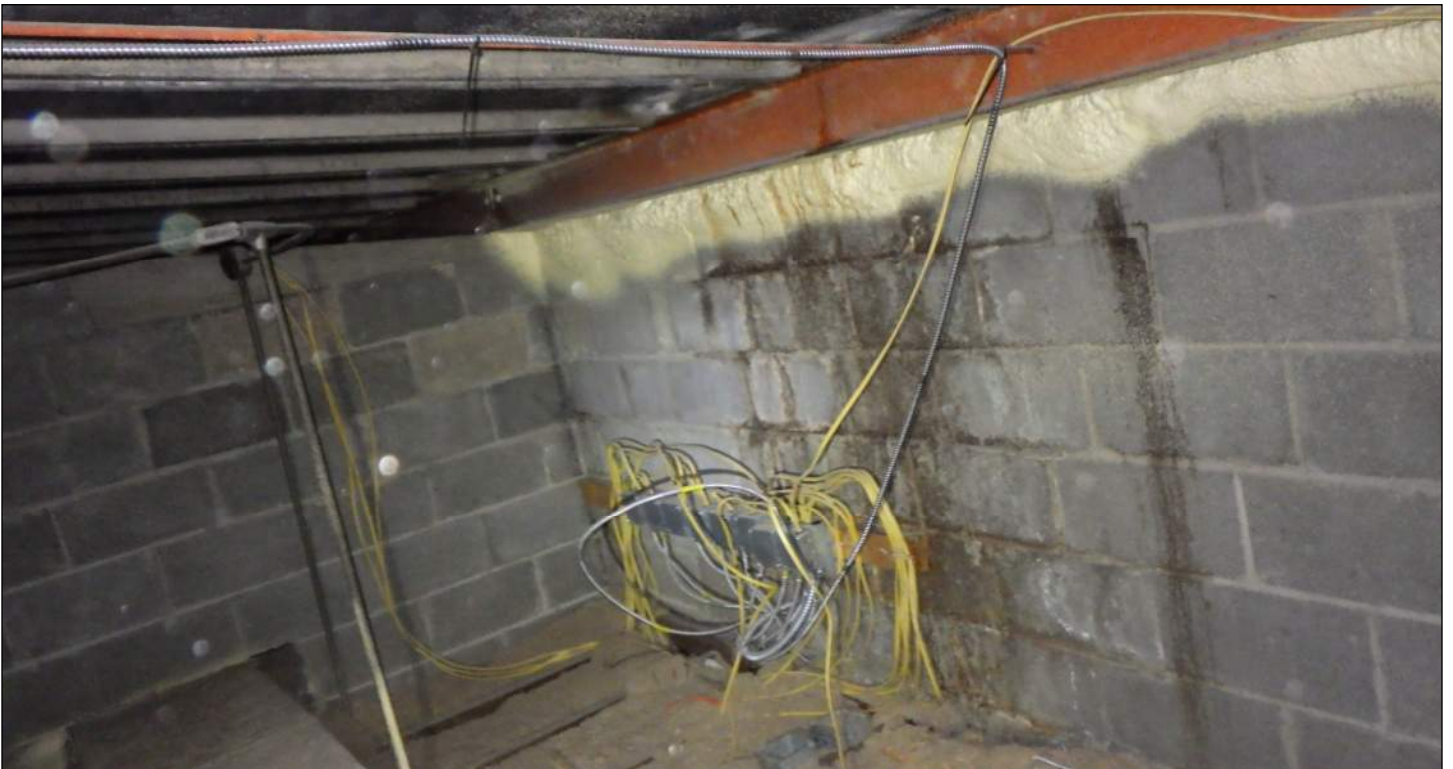
Photo 34: Moisture staining on CMU along south wall of attic.
