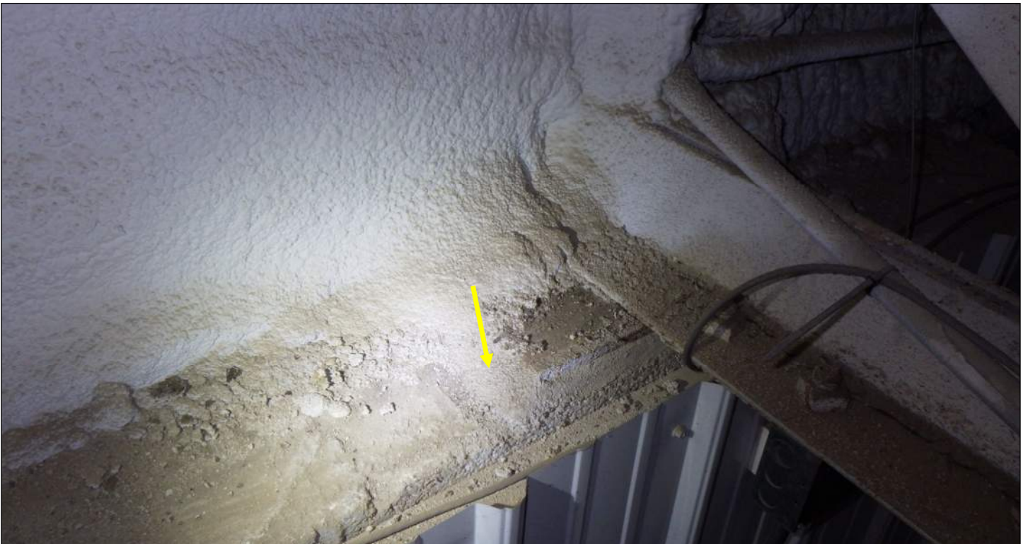
Photo 54: CMU pilaster (arrow) at truss bearing location.
