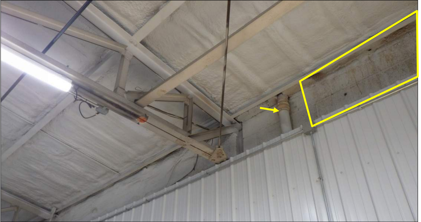
Photo 59: Moisture staining on north CMU wall (box outline), adjacent to roof drain (arrow).
