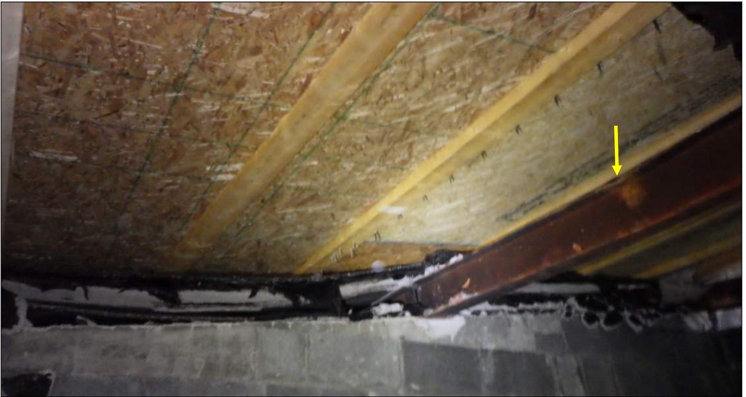
Photo 31: Bent/twisted S7x9.8 beam under area of displaced concrete roof panels.
