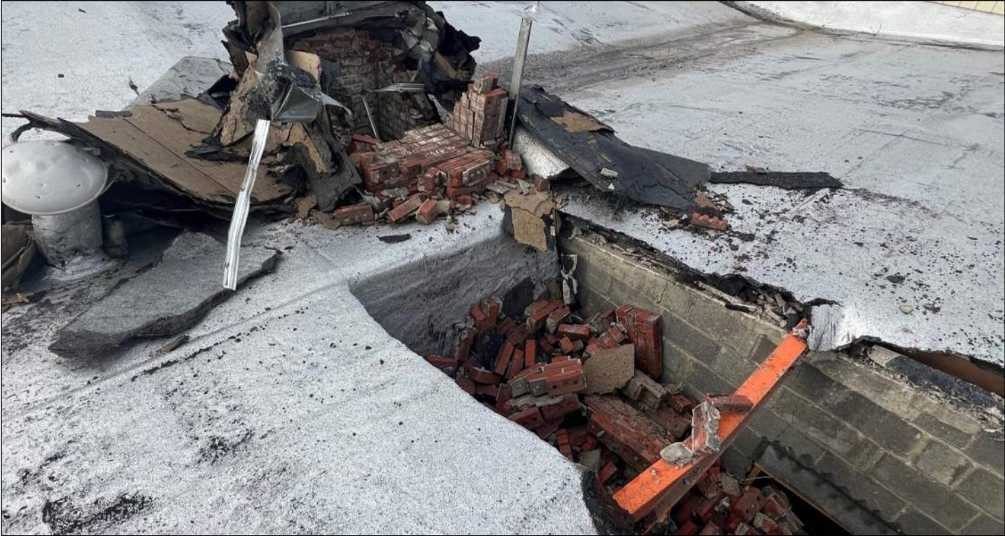
Image 5: Closeup of roof storm damage.
