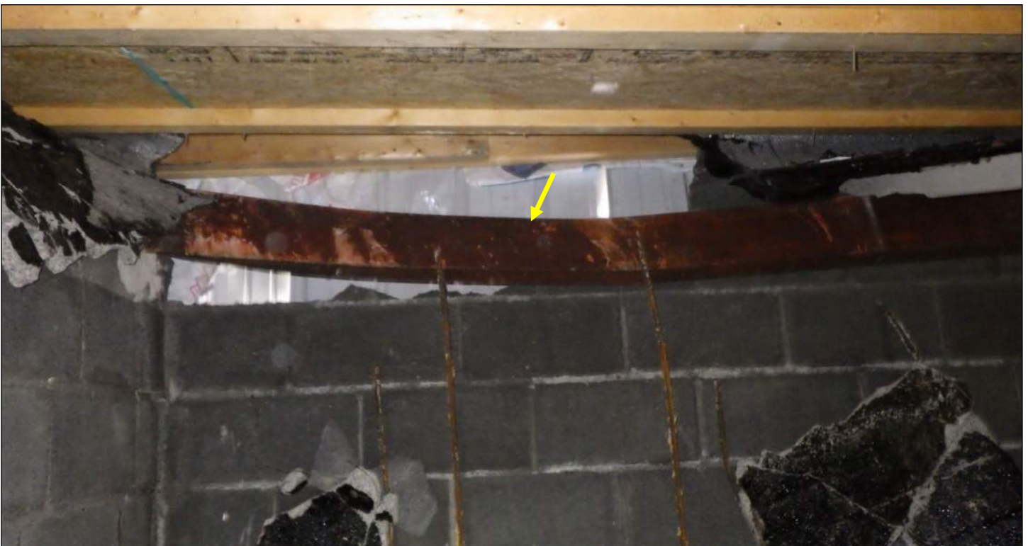
Photo 32: Bent/twisted C7x9.8 beam (arrow) along north exterior CMU wall. Also note fractured/displaced CMU behind damaged beam.
