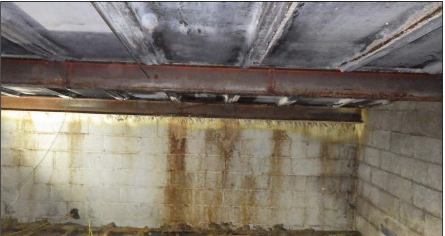
Photo 28: Moisture staining on CMU along south wall of attic. View looking south.
