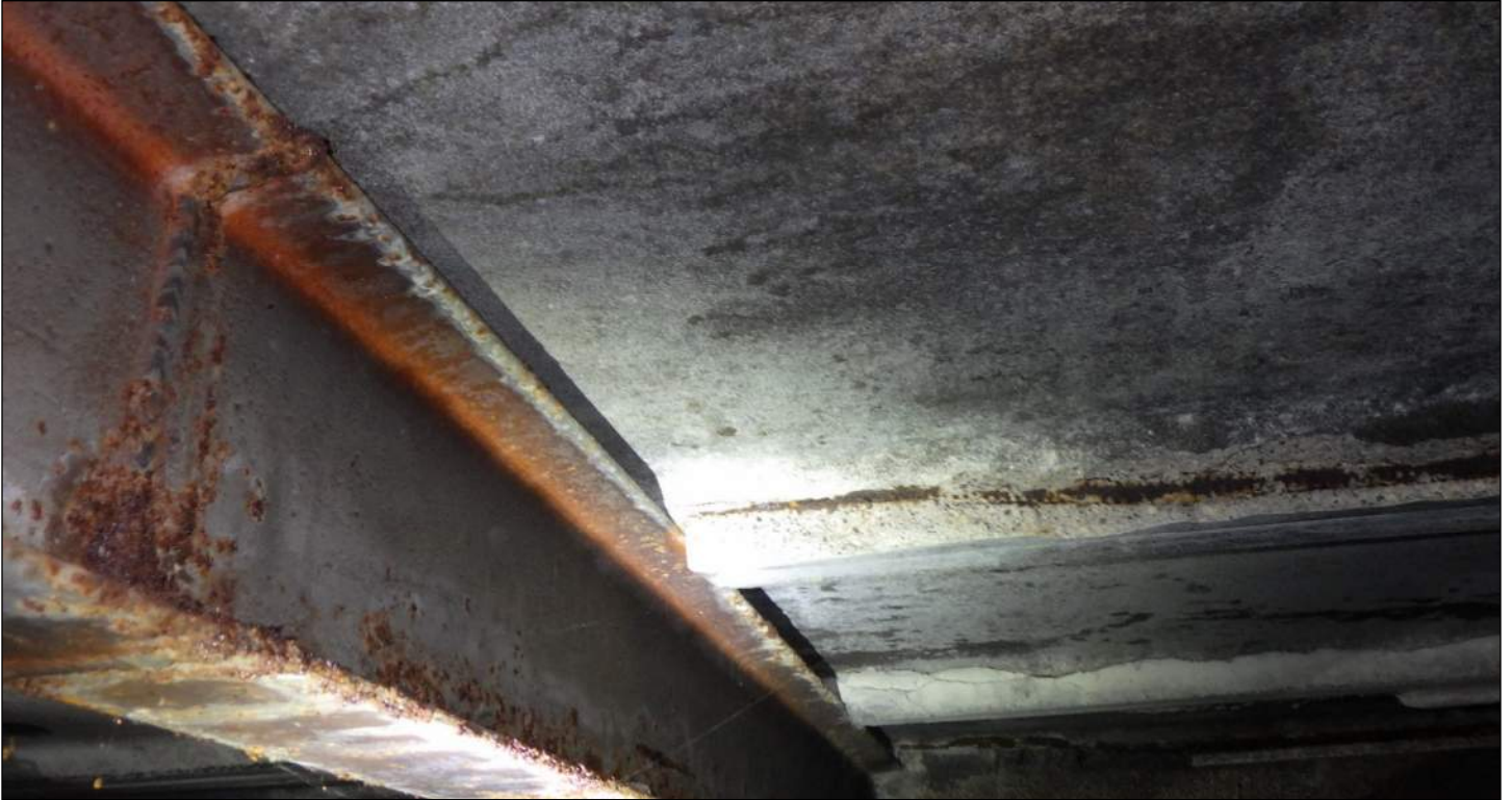
Photo 25: Corrosion of S7x15.3 beam.
