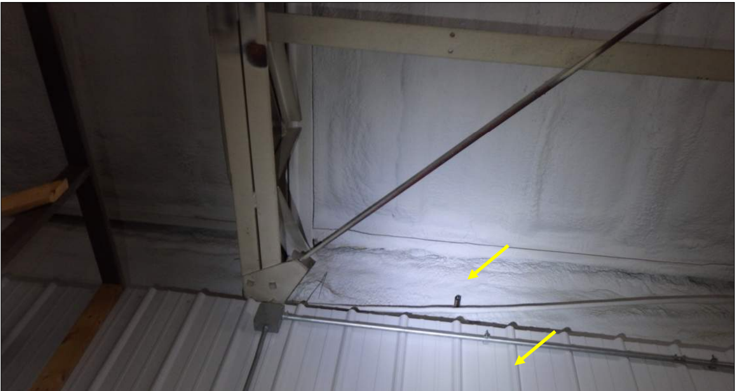
Photo 52: North CMU wall clad with metal panels (bottom arrow) and coated with spray foam (top of photo).
