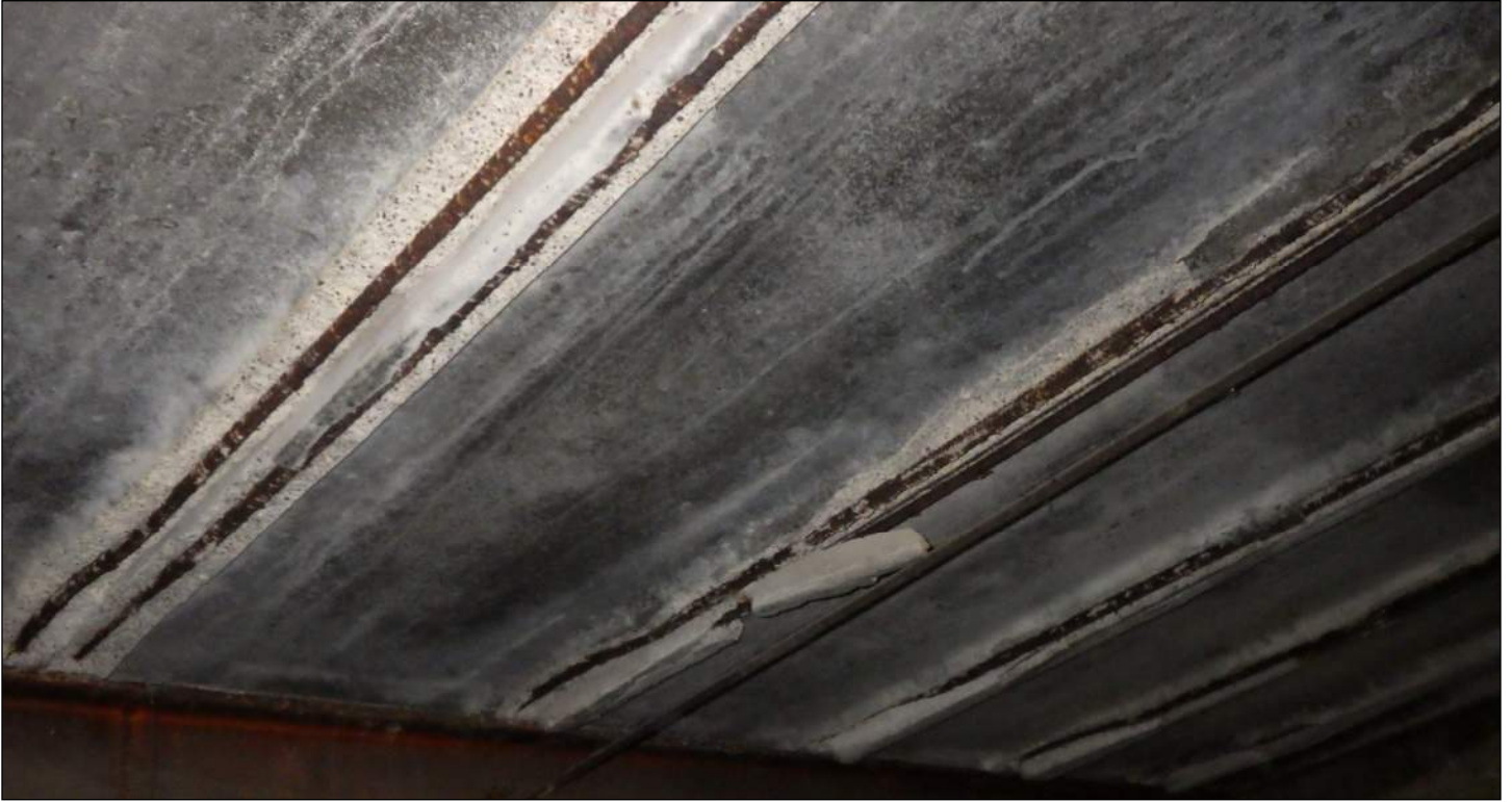
Photo 23: Spalled concrete along flanges of C-shaped precast concrete roof panels. Note moisture stains on panels and visible corrosion of exposed steel reinforcing along flanges.
