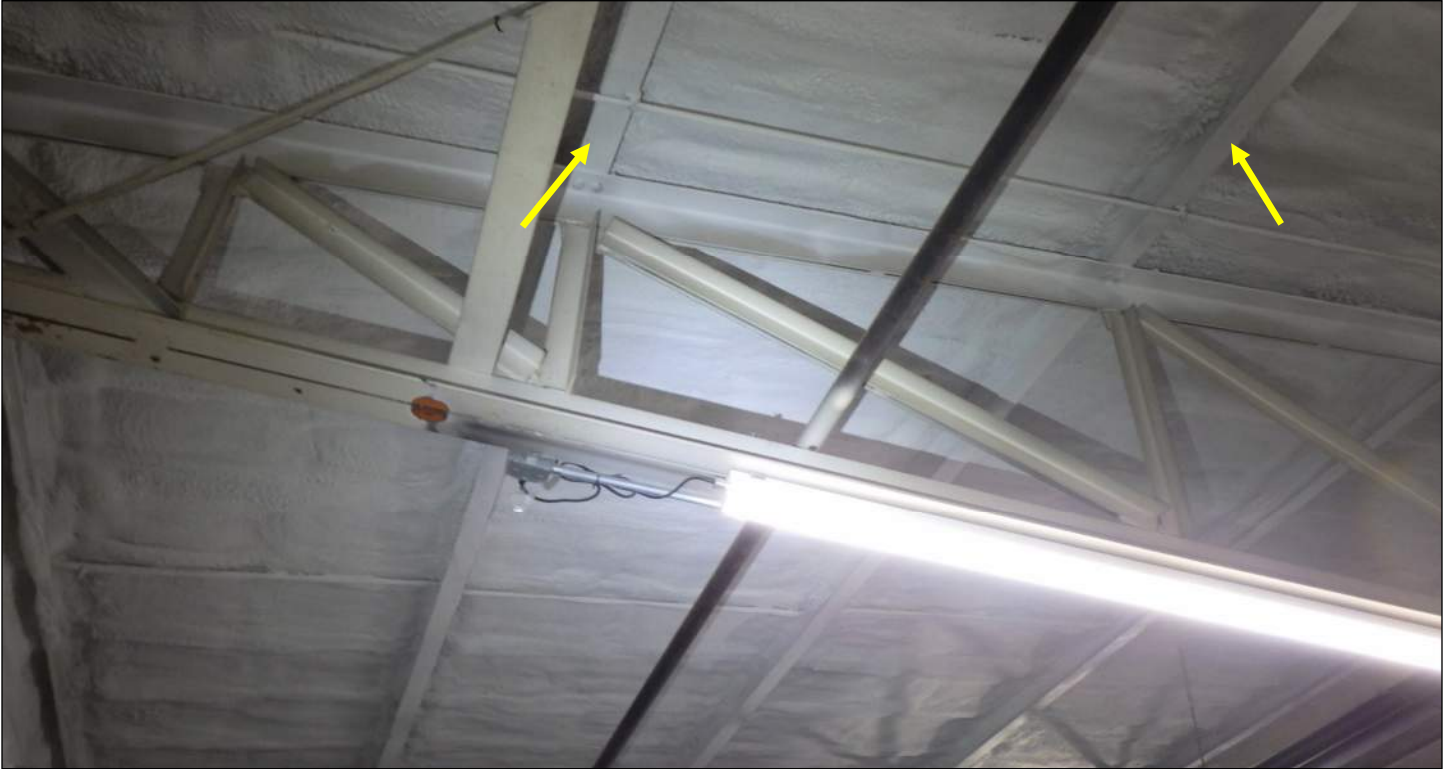
Photo 51: Roof beams (arrows) spanning between trusses.
