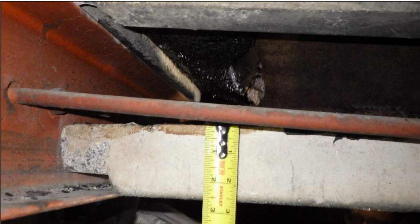
Photo 20: Side view of typical precast concrete roof panel. Note this panel in Bay 2 had partially collapsed.
