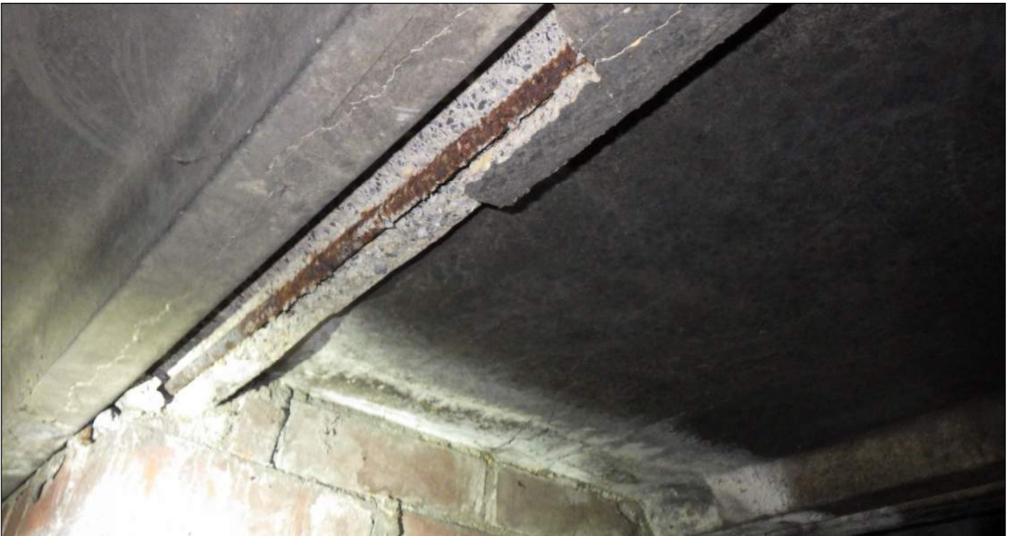
Photo 30: Spalled and cracked concrete along flanges of C-shaped precast concrete roof panels. Note moisture stains on panels and visible corrosion of exposed steel reinforcing along flange.
