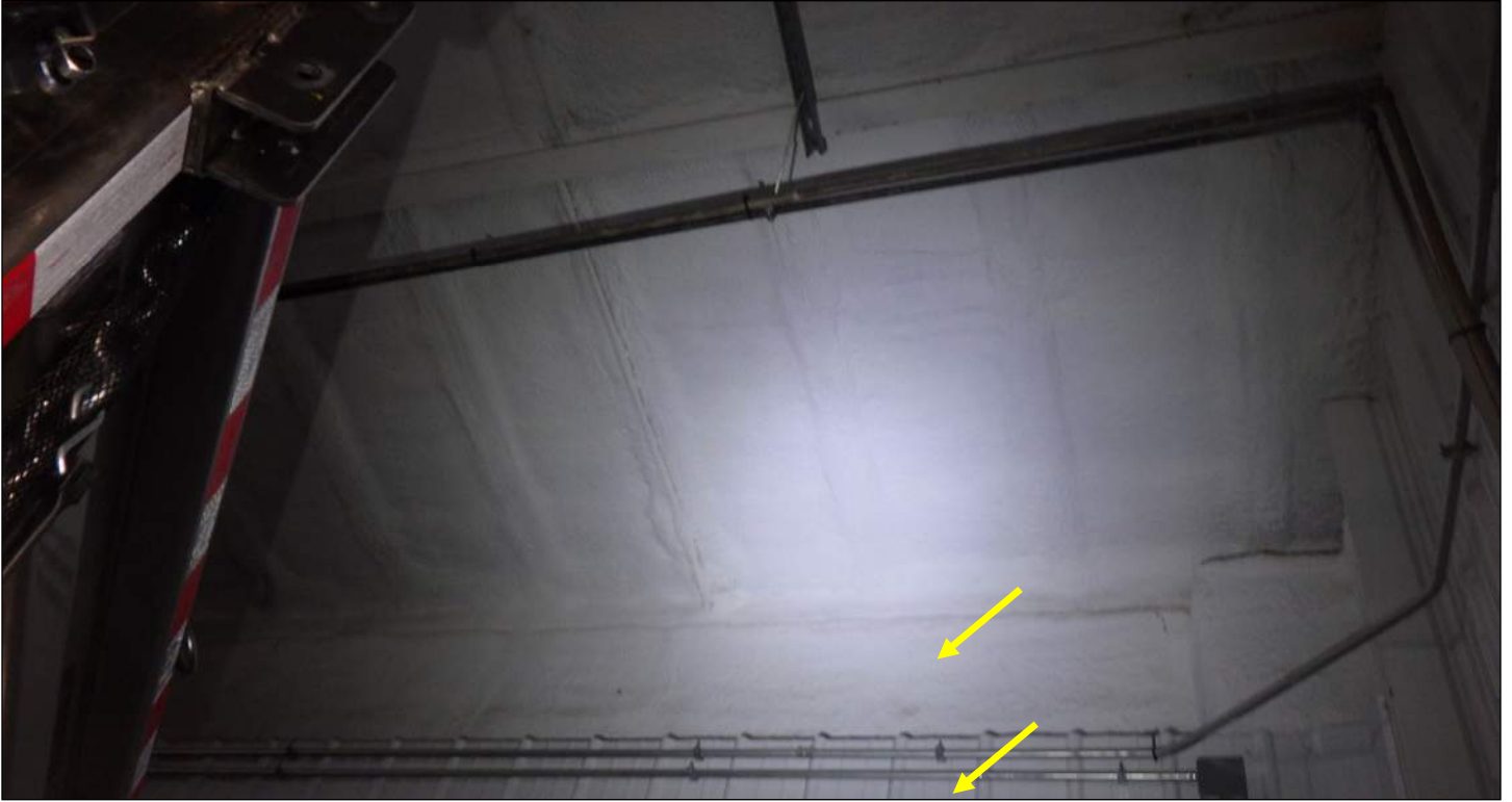
Photo 53: South CMU wall clad with metal panels (bottom arrow) and coated with spray foam (top of photo).
