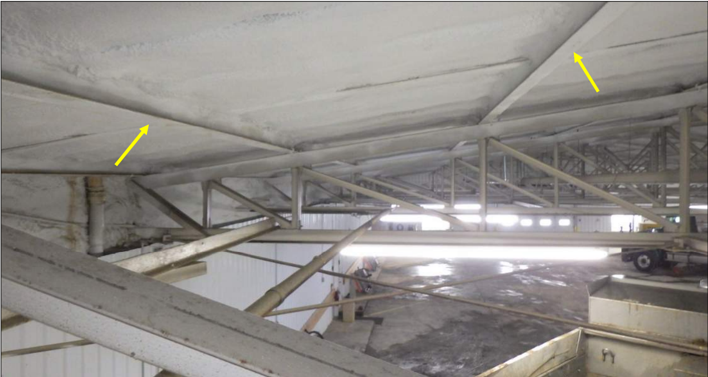
Photo 50: Roof beams (arrows) spanning between trusses.
