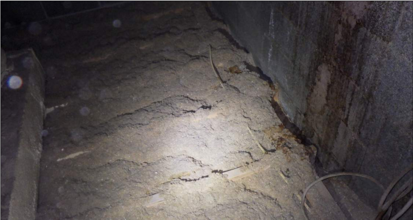
Photo 38: Moisture staining on CMU along south wall of attic.
