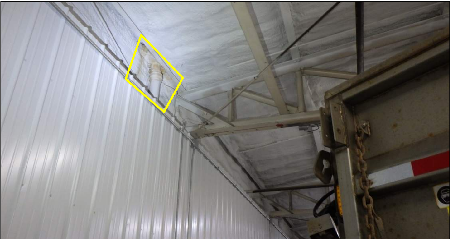
Photo 60: Moisture staining on north CMU wall (wall coated in spray foam) at roof drain.
