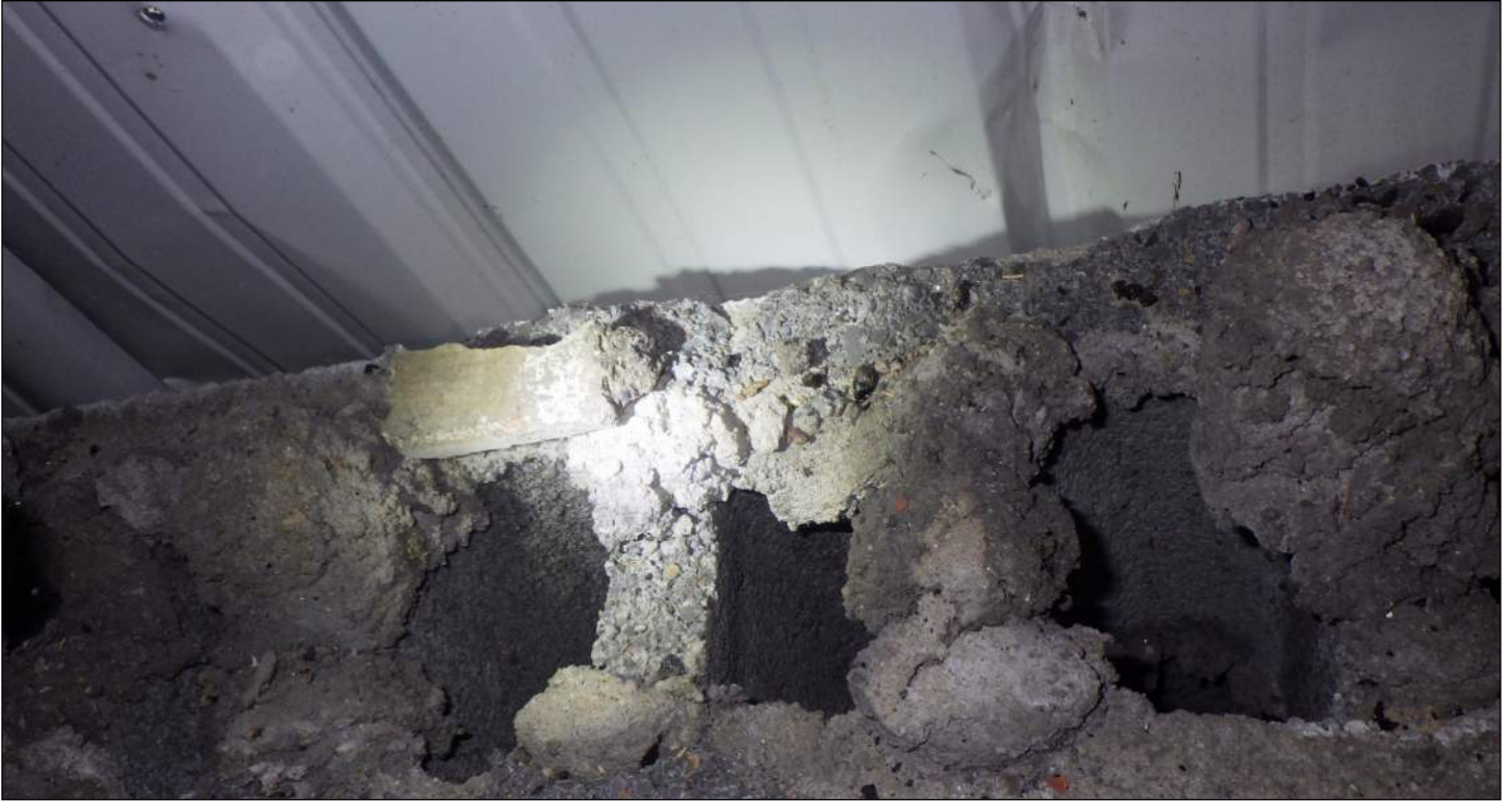
Photo 21: View looking downward at CMU along north wall of Bay 1. Note top of CMU is visible due to CMU displaced as result of storm/impact damage. Also note CMU is hollow and unreinforced.
