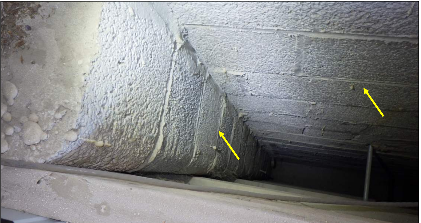
Photo 56: CMU pilaster (left arrow) within CMU wall (right arrow). View from above looking downward.
