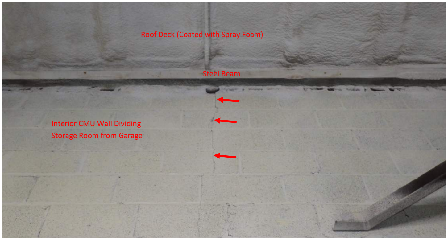
Photo 45: Overview of east storage room, looking up and to the south. Note vertical crack in CMU (arrows). Also note moisture stains on roof and rust spots on steel roof beam.
