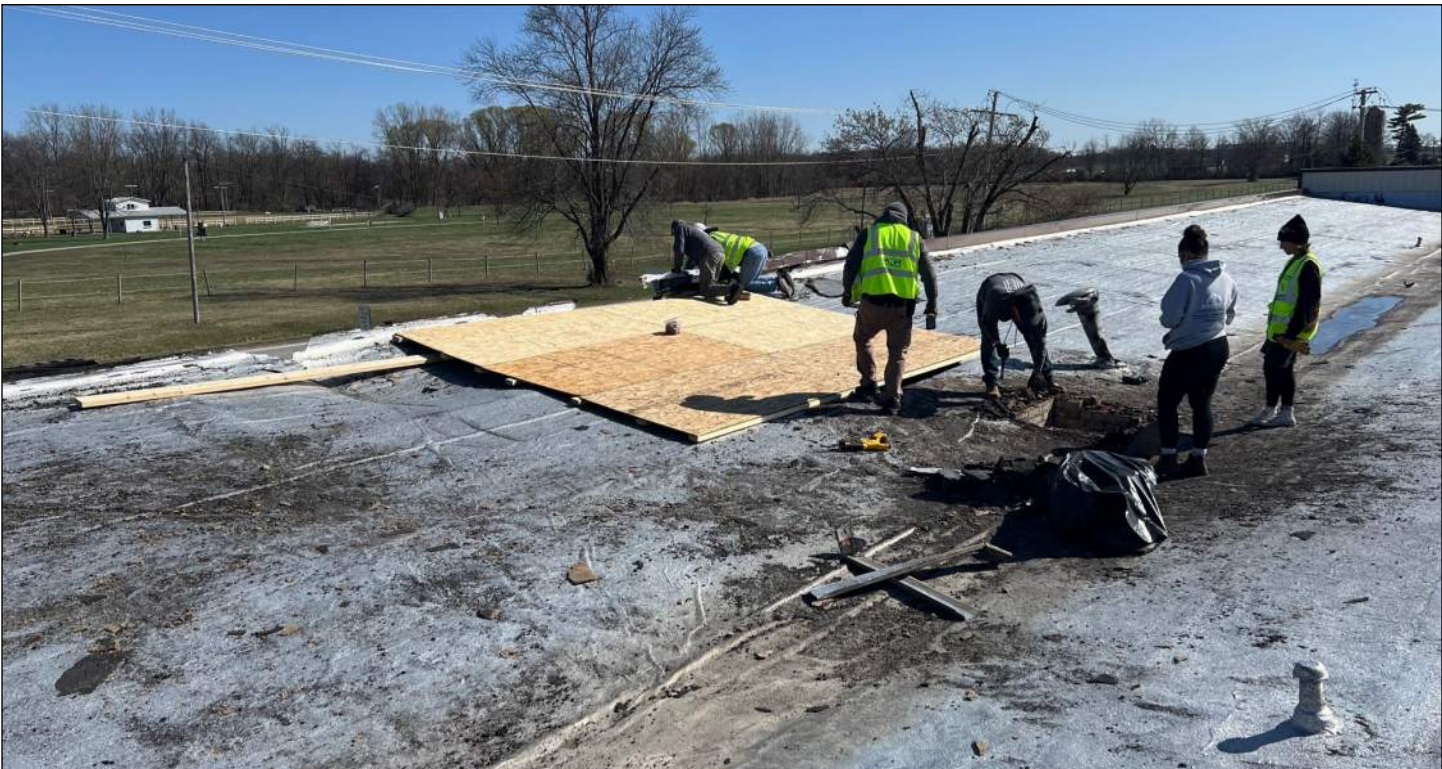
Image 6: Overview of roof during installation of temporary covering.
