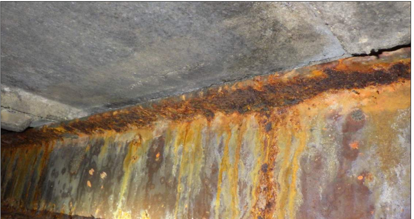
Photo 26: Corrosion of S7x15.3 beam.
