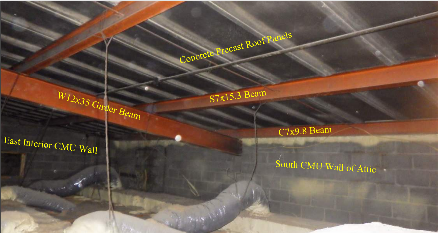
Photo 18: Overview of roof framing in Bay 3.
