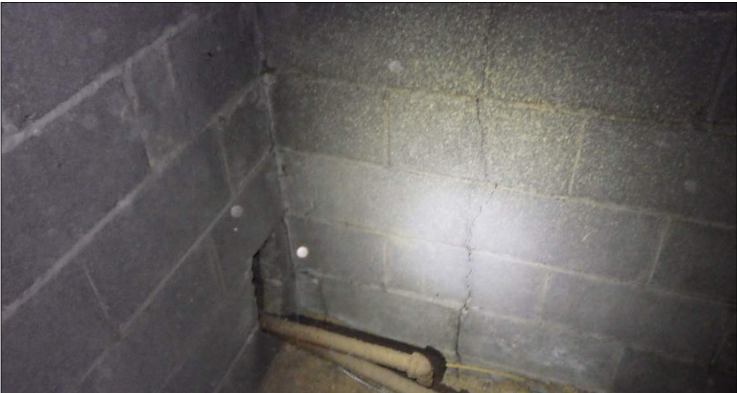
Photo 36: Vertical crack in CMU along north exterior wall.
