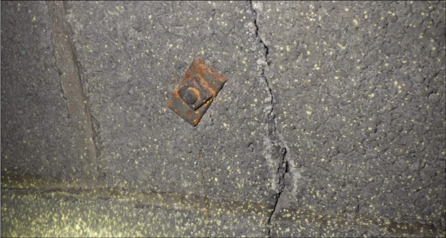
Photo 37: Closeup of crack in CMU shown in previous view.
