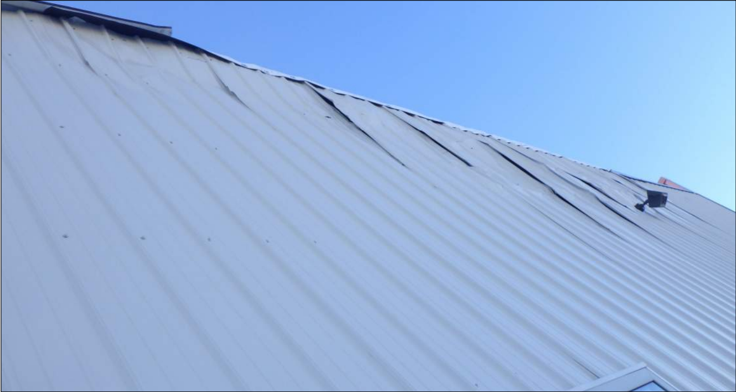
Photo 7: Closeup of storm/impact damaged siding near west end of north elevation.
