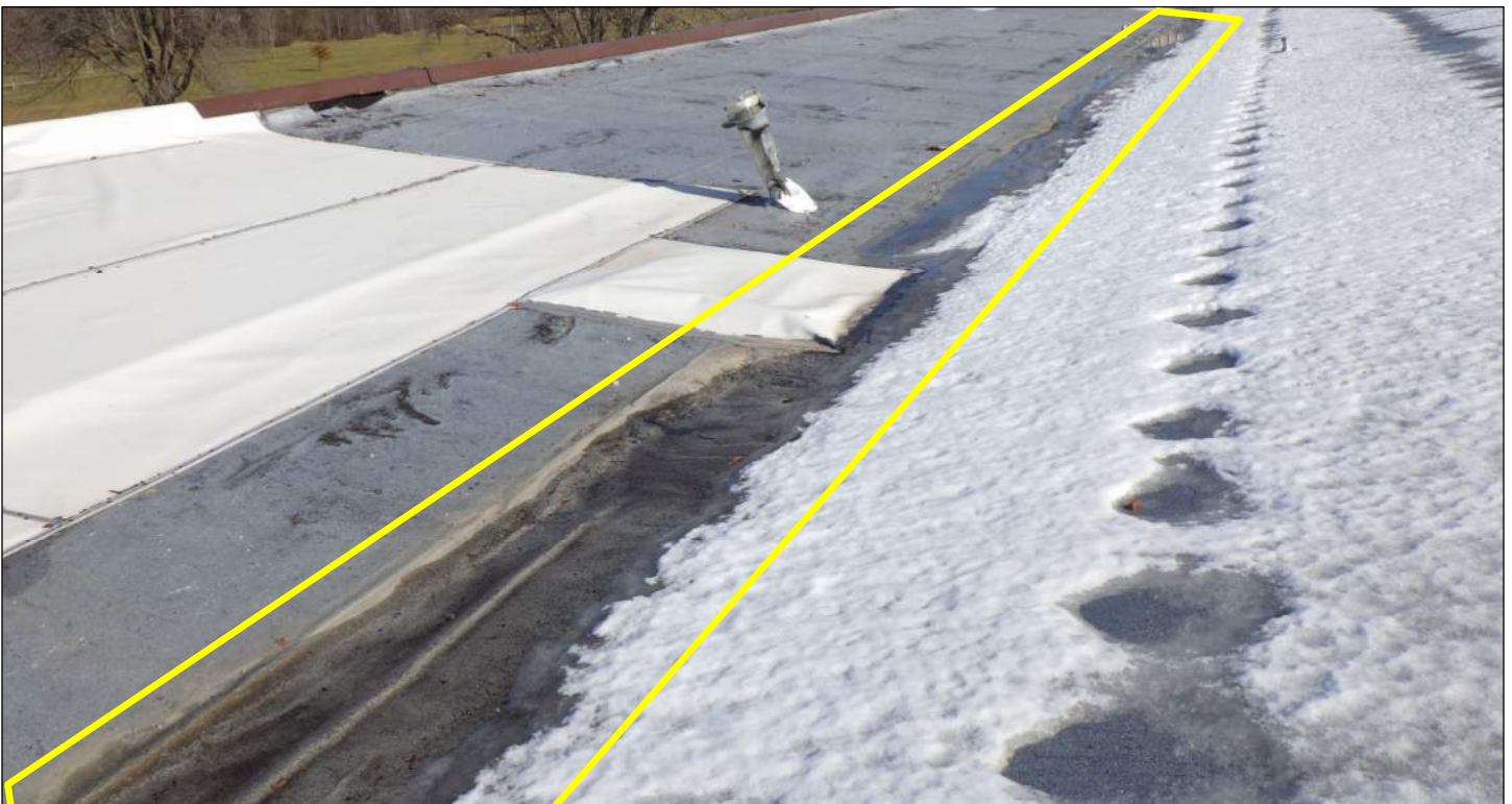
Photo 14: Standing water (boxed outline) in valley between roof over office area (left in photo) and roof over garage area (right in photo).
