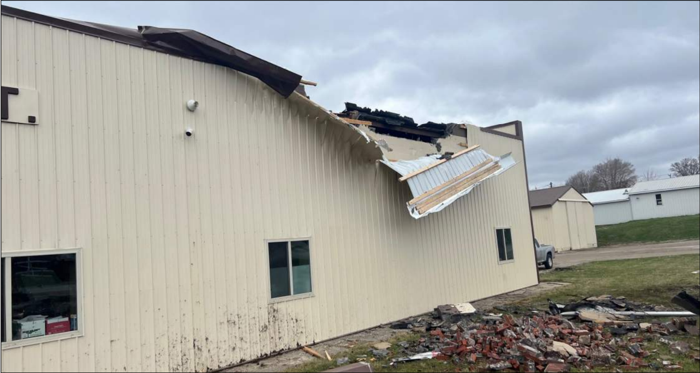
Image 3: Closeup of north wall storm damage.
