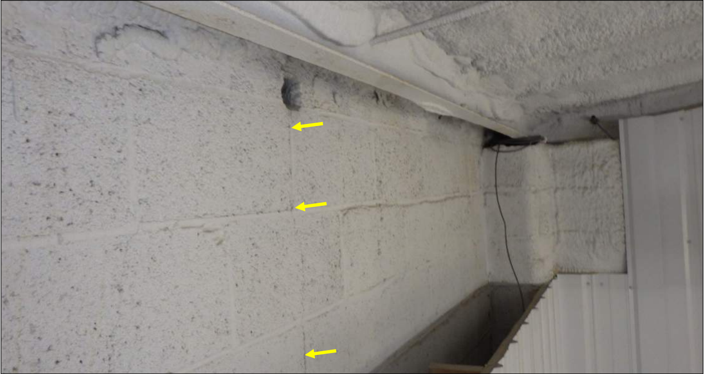
Photo 57: Overview of CMU wall section above metal panels. Note thin vertical crack in CMU that aligns with crack on other side of wall in east storage room (reference Photo 45).
