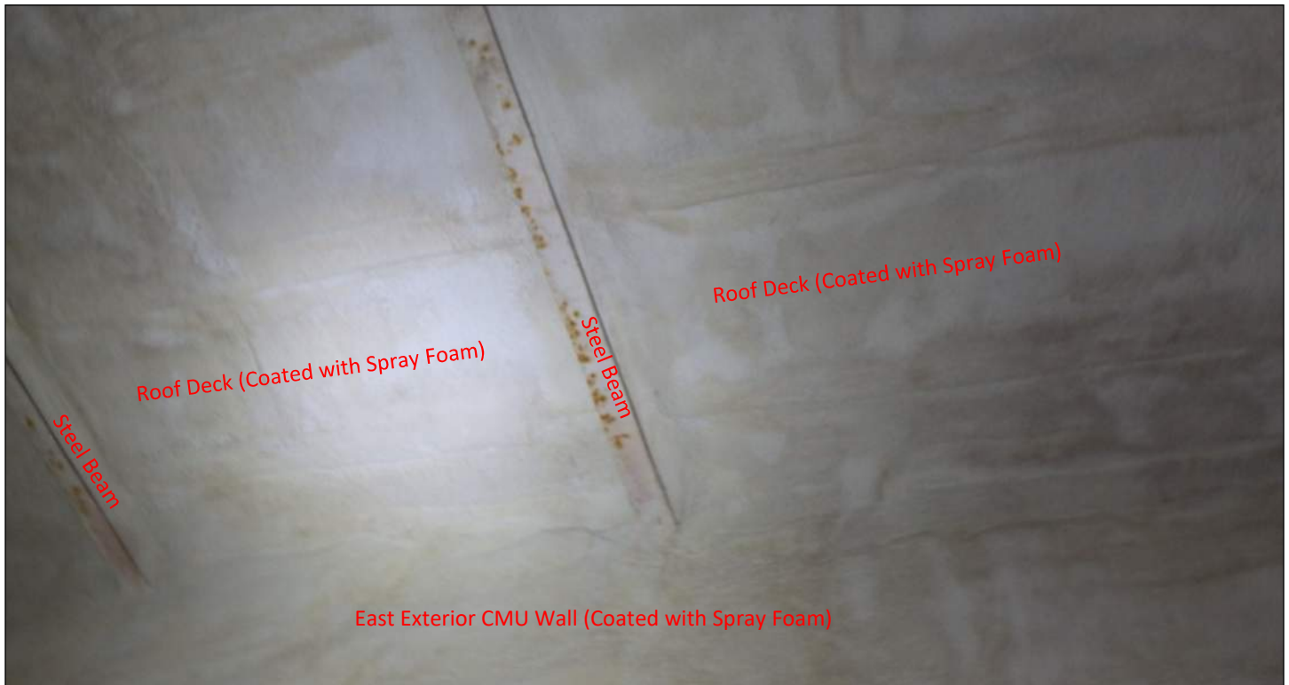
Photo 43: Overview of east storage room, looking up and to the east. Note moisture stains on roof deck and north CMU wall. Also note rust spots on steel roof beam.
