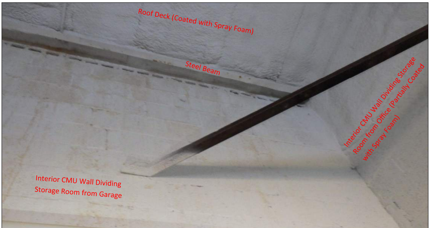
Photo 44: Overview of west storage room, looking up and to the southwest. Note moisture stains on south CMU wall. Also note rust spots on steel roof beam.
