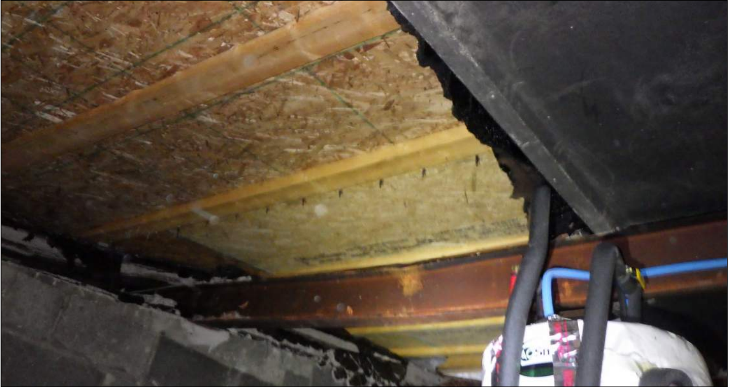
Photo 29: Overview of temporary oriented strand board covering installed over area of roof panels fractured/displaced by impact from chimney.
