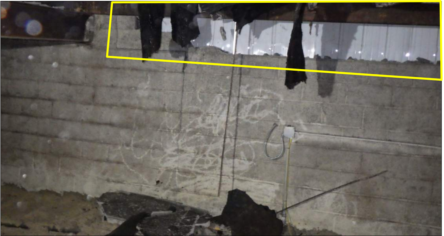
Photo 27: Fractured/displaced CMU along north wall.
