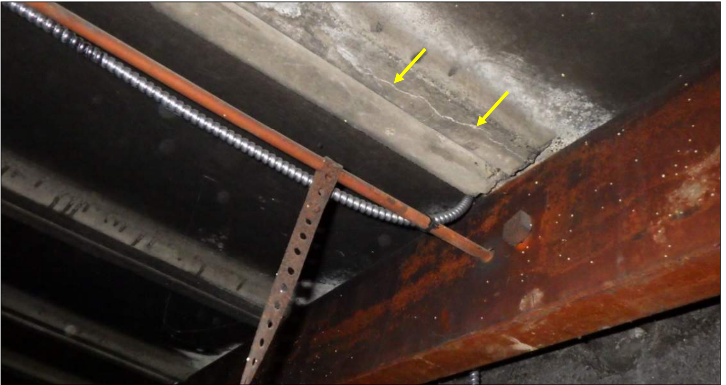
Photo 33: Crack in flange of roof panel (arrows). Also note moisture stains on panel.
