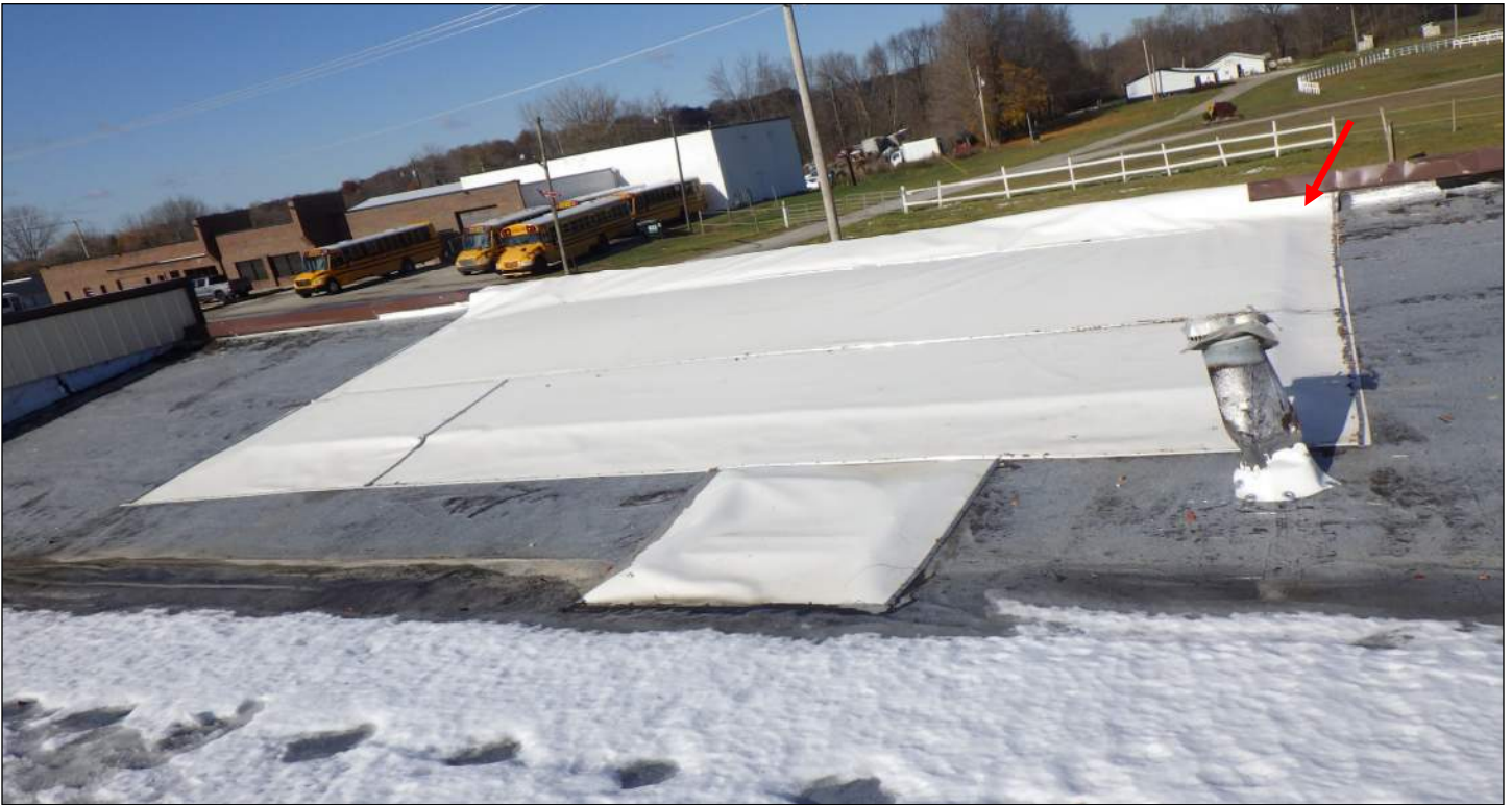
Photo 13: Temporary covering installed over roofing.
