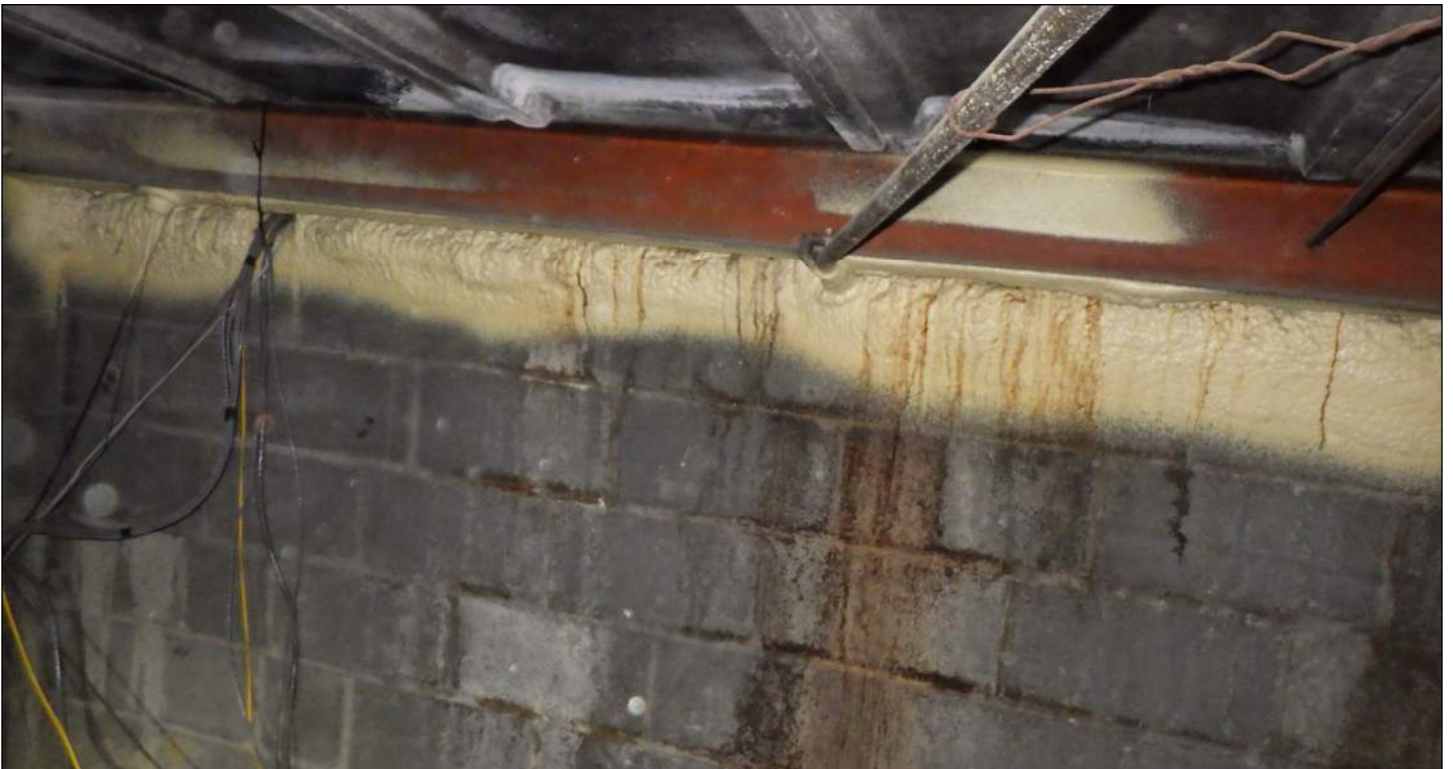
Photo 40: Moisture staining on CMU along south wall of attic.
