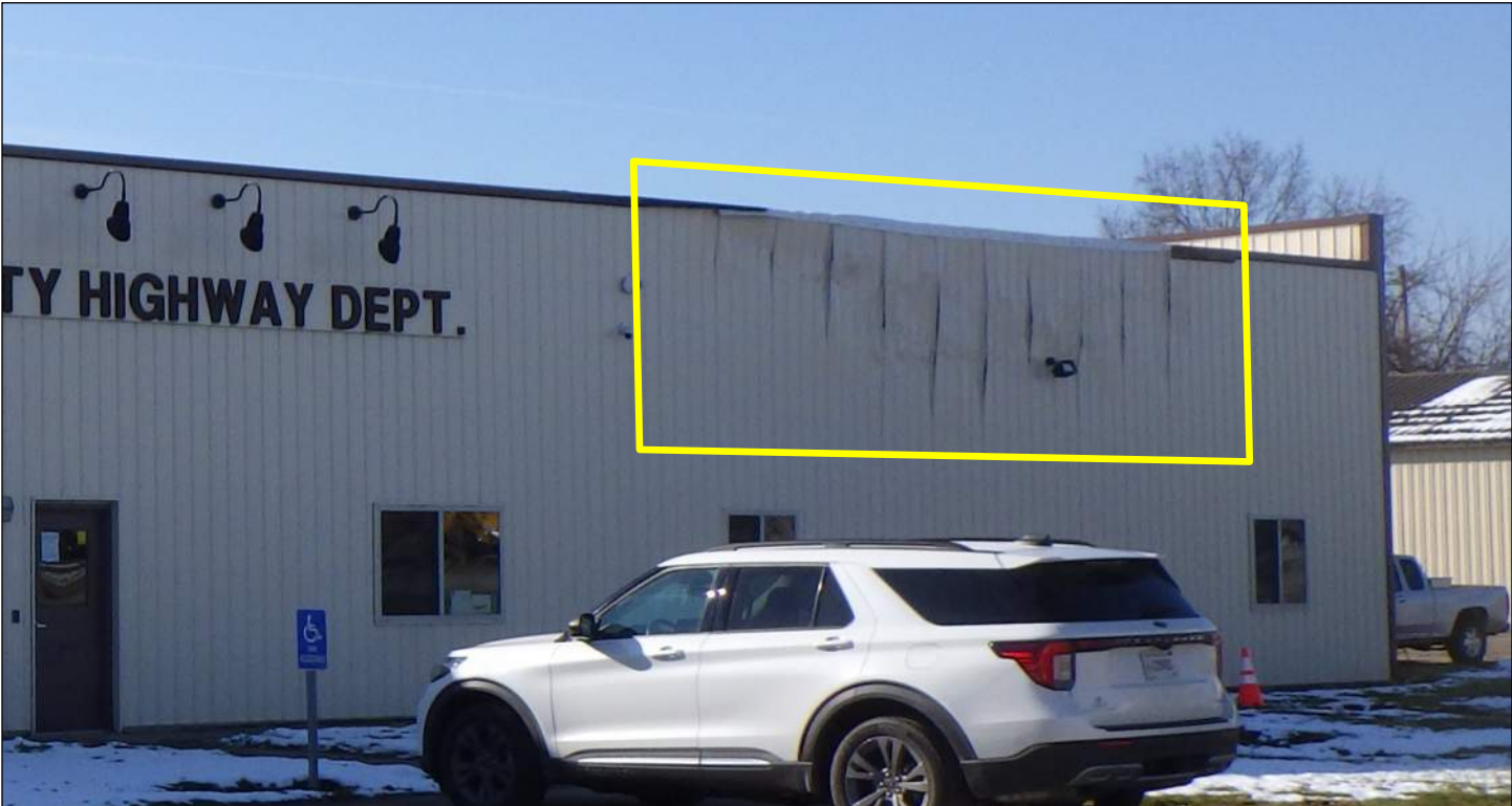
Photo 6: Storm/impact damaged siding on north elevation.
