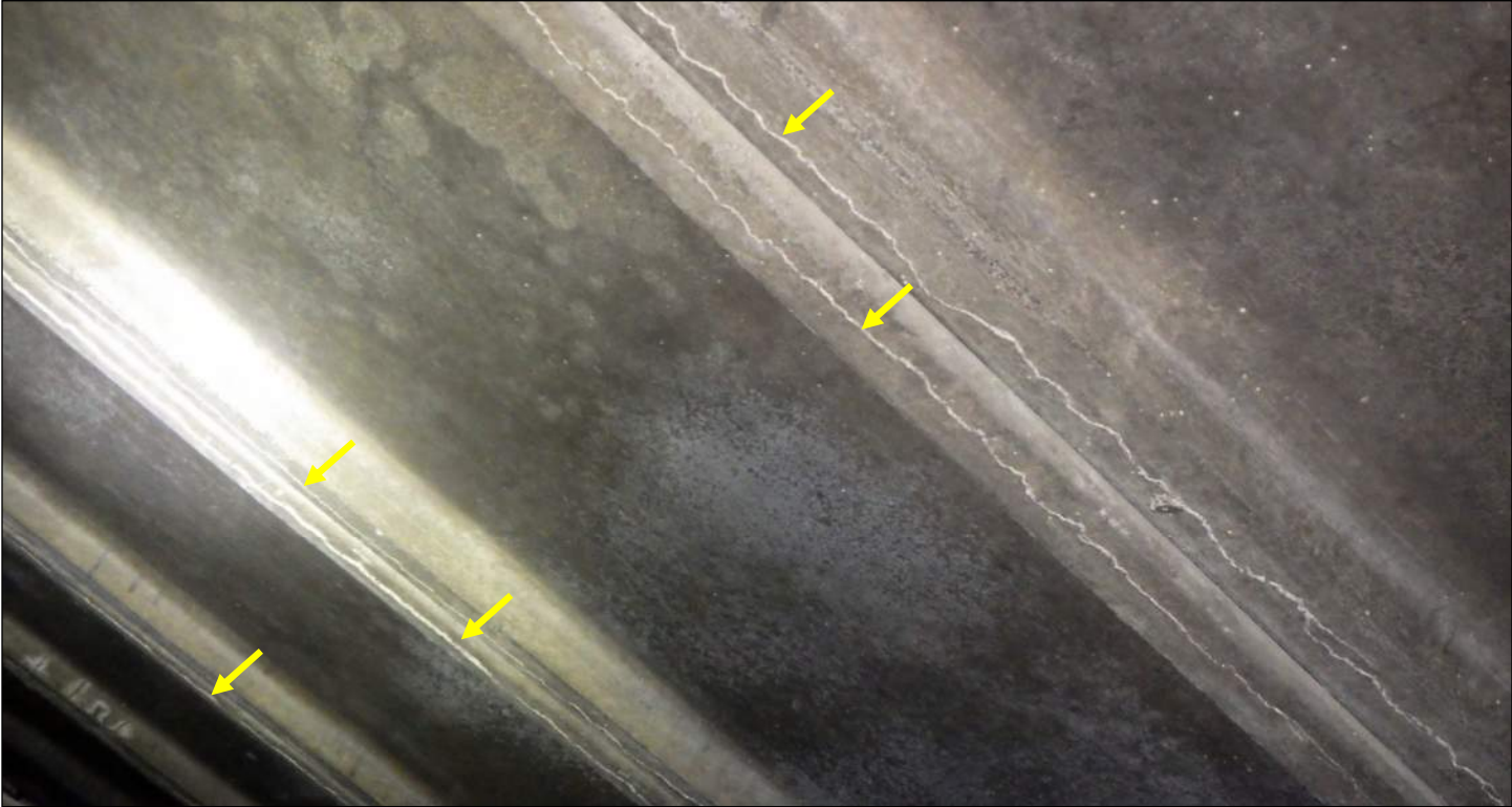
Photo 35: Cracks in flanges of roof panels.
