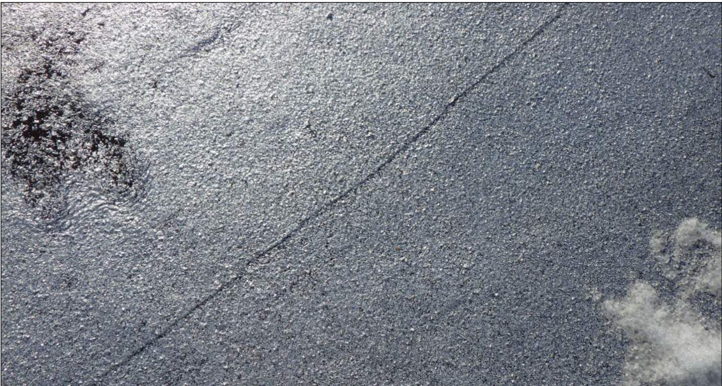
Photo 12: Closeup of aluminum chip top coating on roofing.
