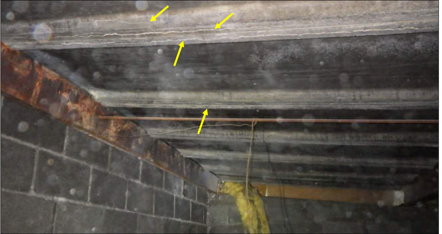
Photo 39: Cracks in flanges of roof panels.
