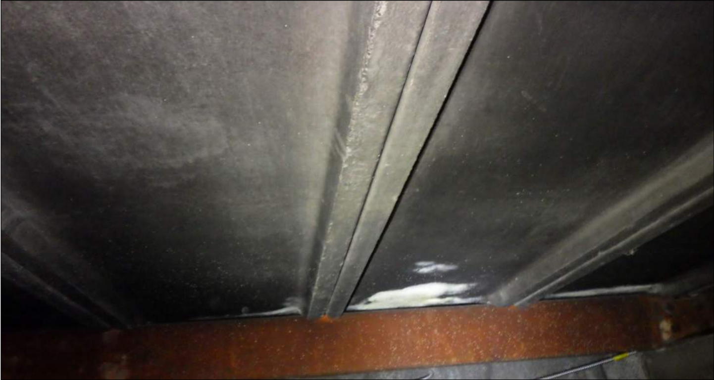
Photo 19: Underside view of typical precast concrete roof panels.
