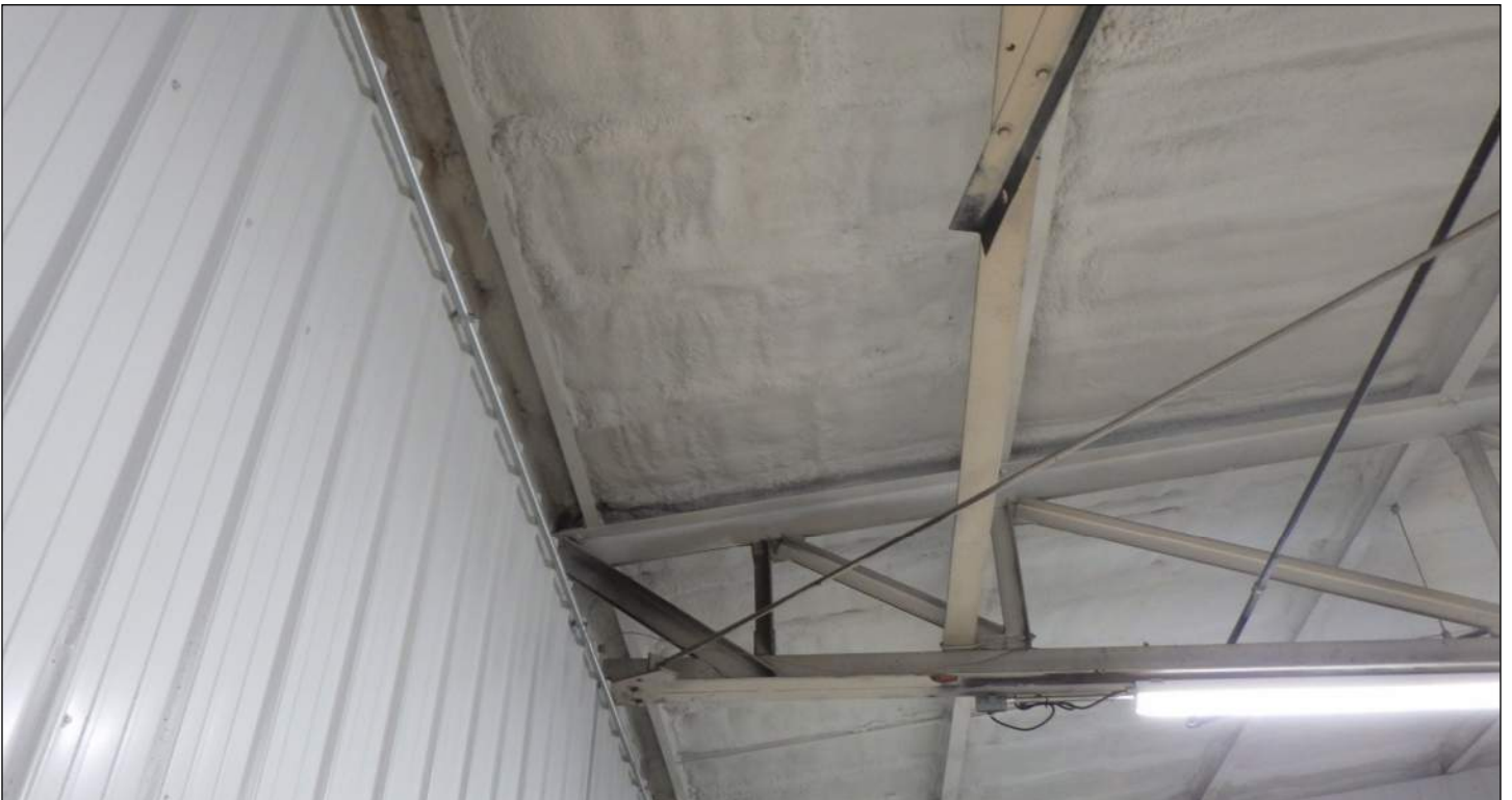
Photo 48: Underside of roof structure along north eave of garage roof (shared valley with office roof).
