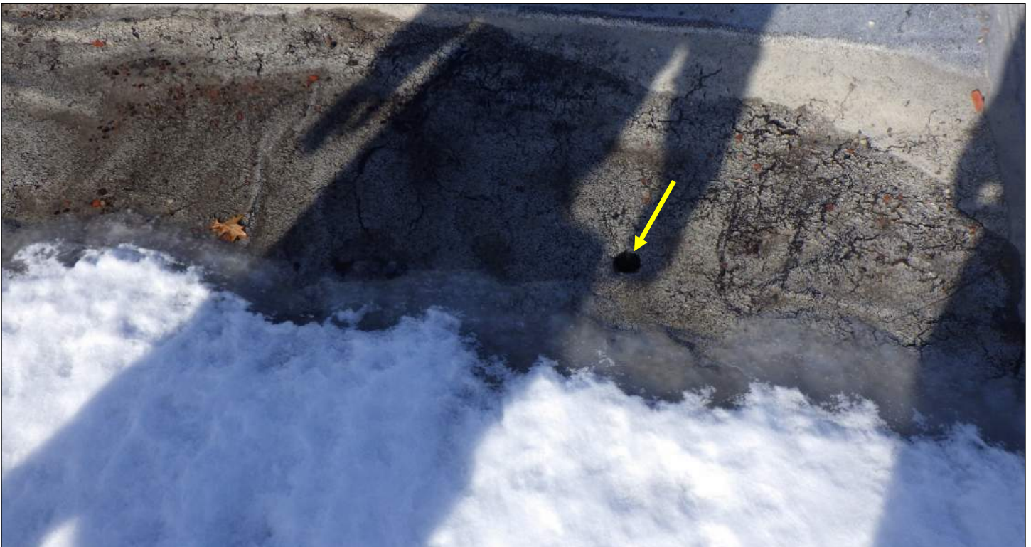
Photo 16: Drain hole in roofing.
