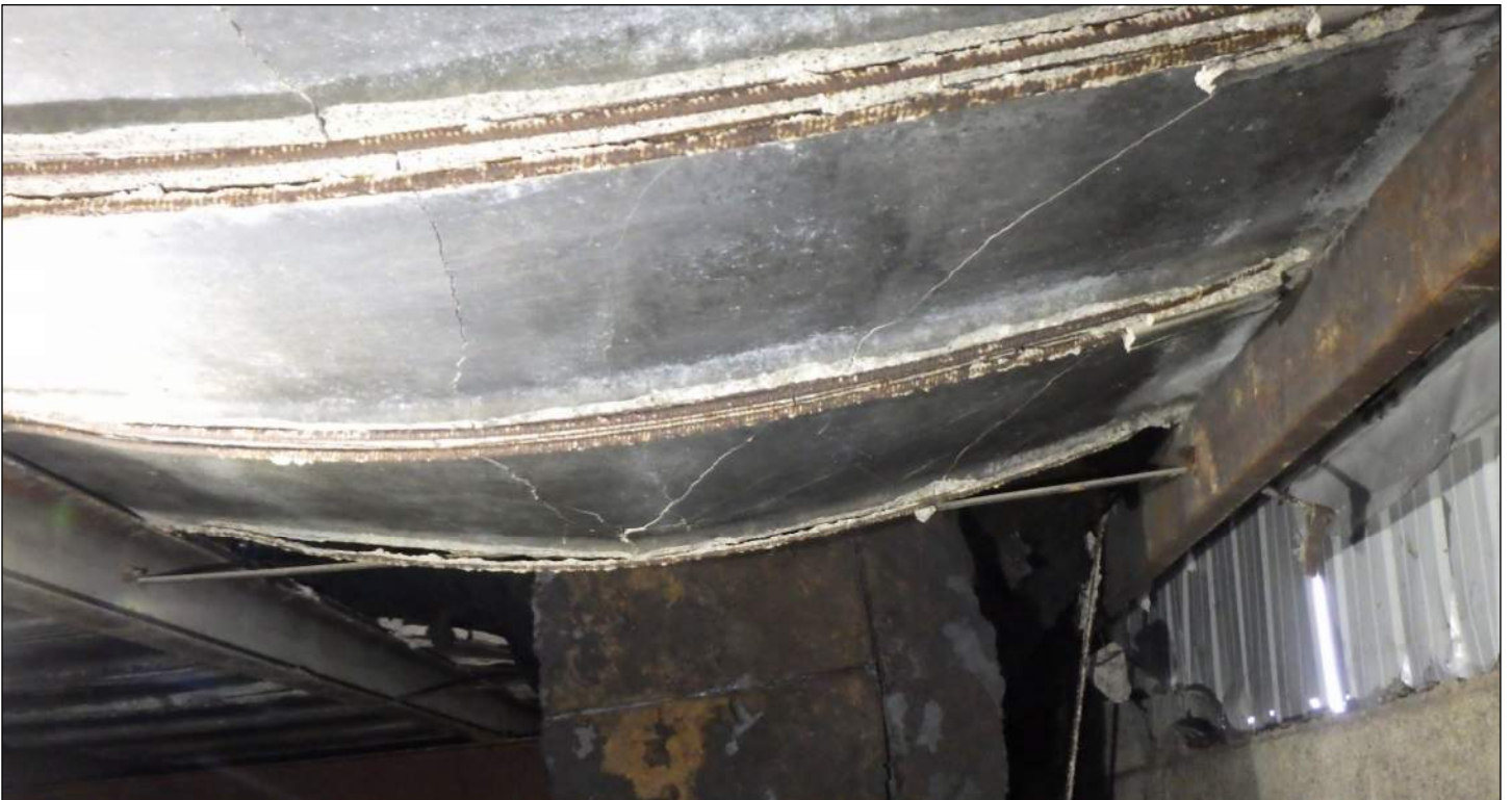
Photo 22: Precast concrete panels in area of chimney impact area. Note panels are deteriorated, cracked, and appear to be in imminent danger of collapse. View looking west.
