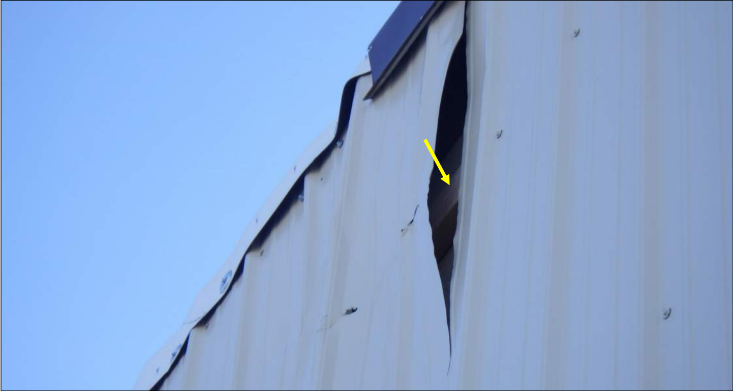
Photo 5: Wood furring strip visible behind area of damaged siding.
