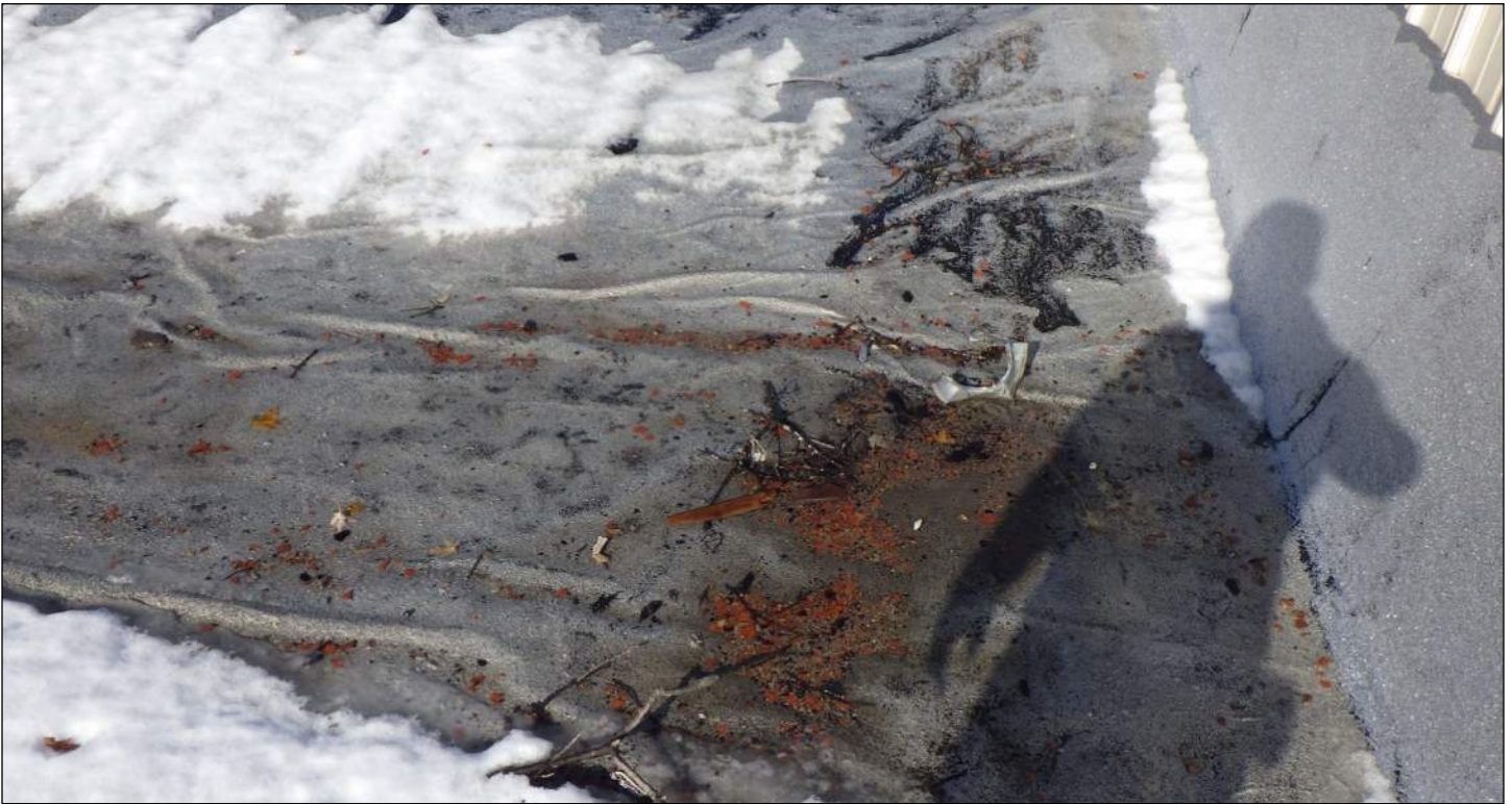
Photo 15: Closeup of standing water in valley at east end of roof.
