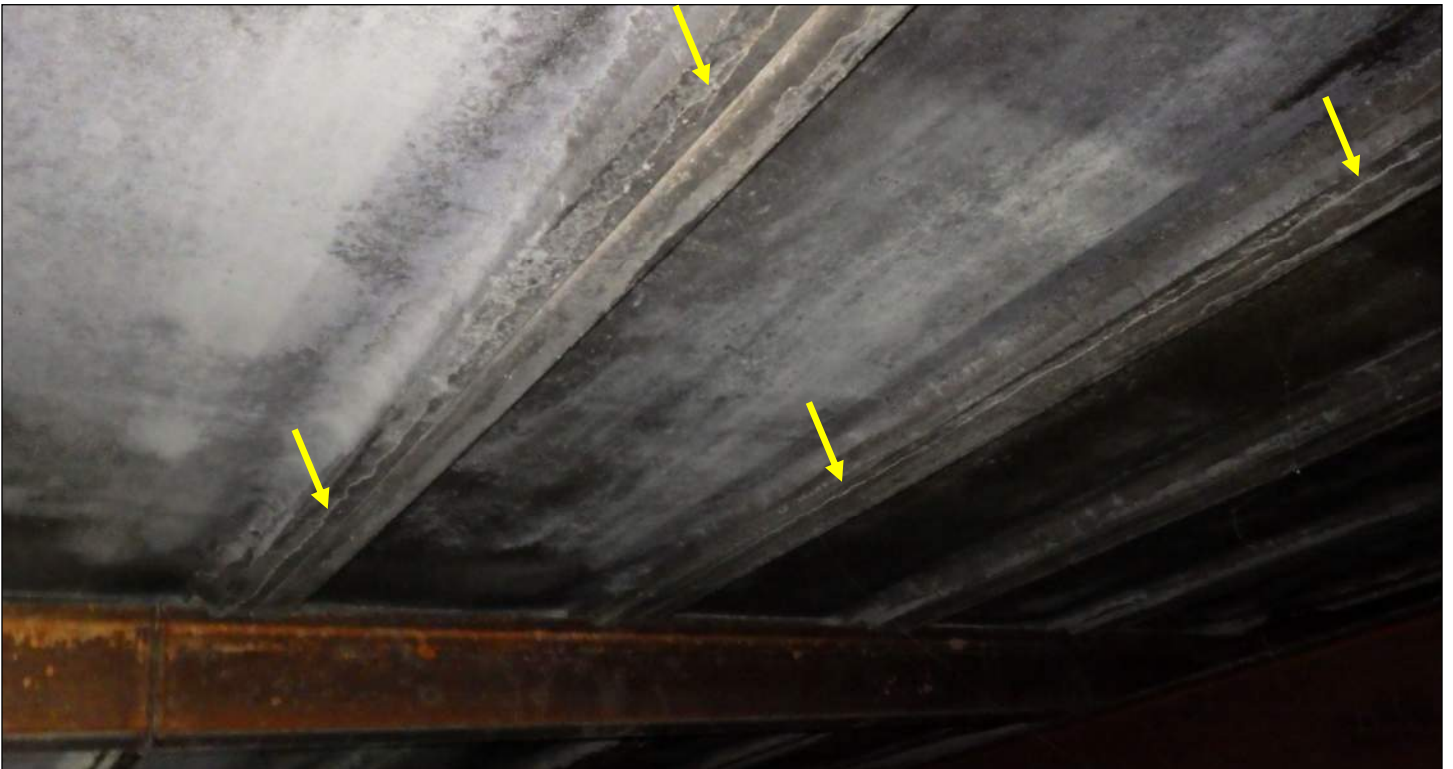
Photo 24: Cracks in flanges of C-shaped precast concrete roof panels.
